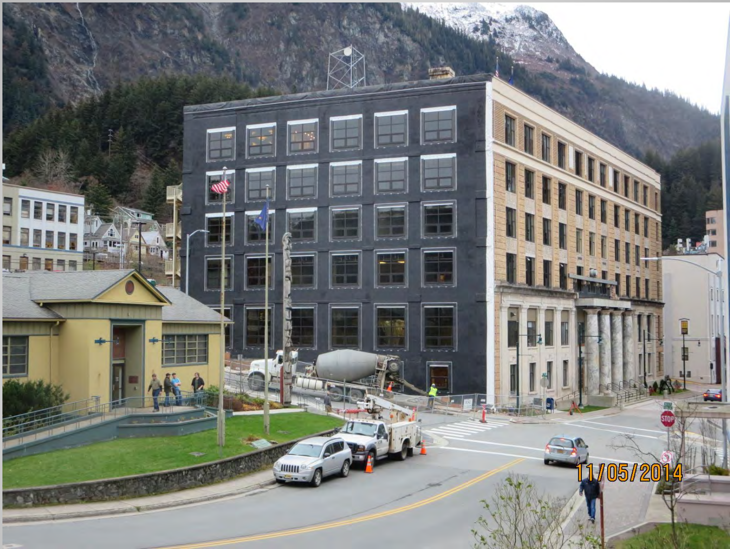
New Windows-Temporary Water Proofing
