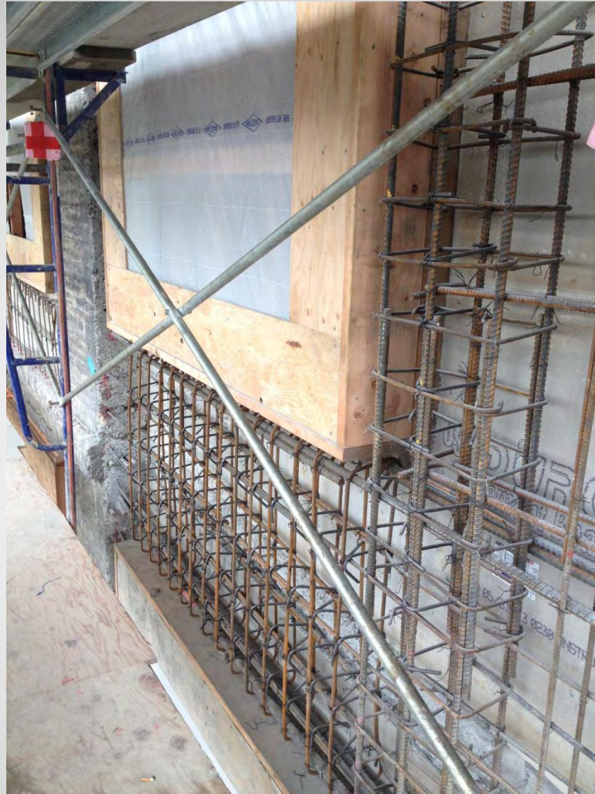
Reinforcing for Shear Wall
