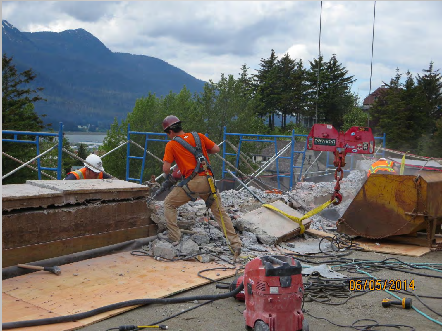
Removing the Parapets
