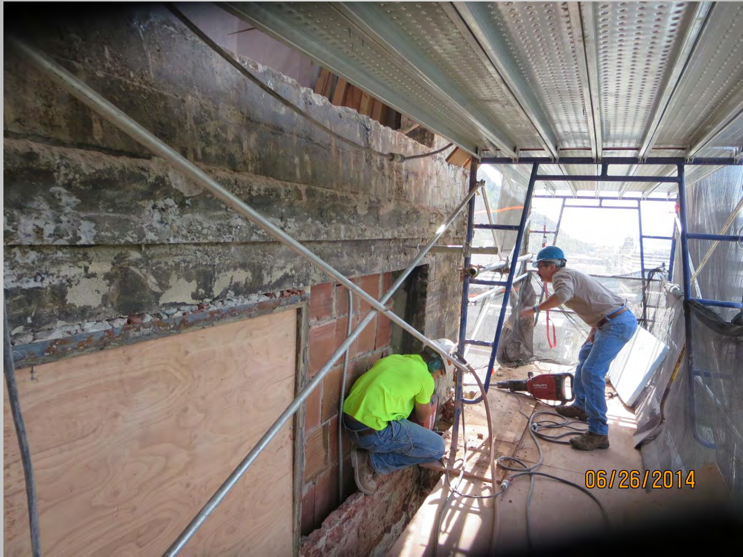
Exterior Demolition 4 th Floor
