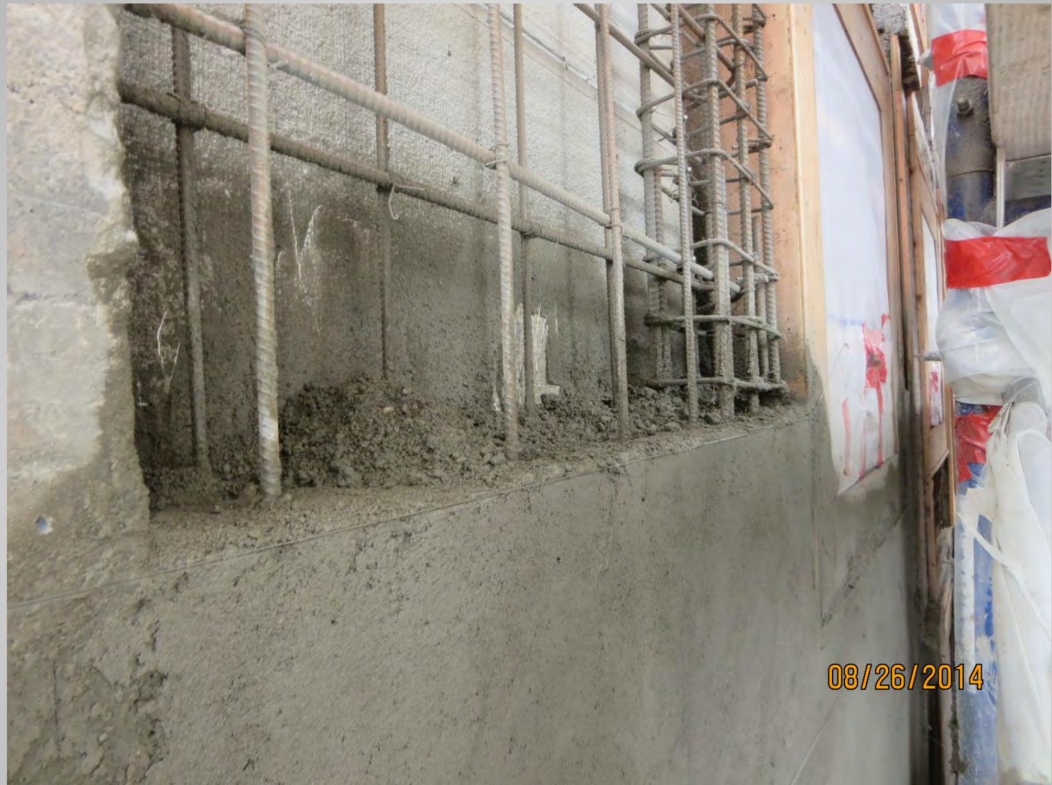
Shotcrete after Screeding
