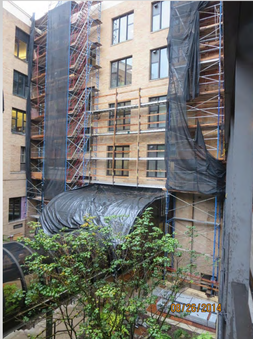
Infill Construction in Courtyard
