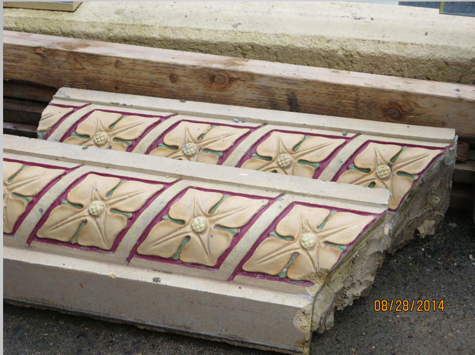
Terracotta Window Surrounds
