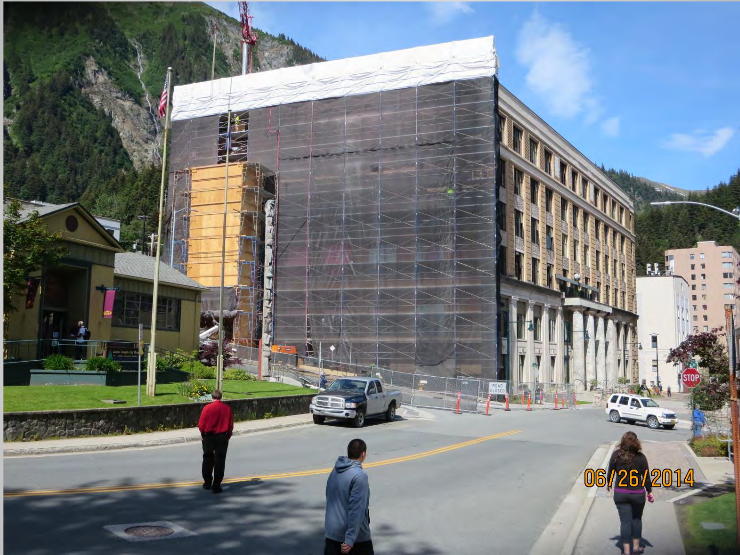
Scaffolding West Side
