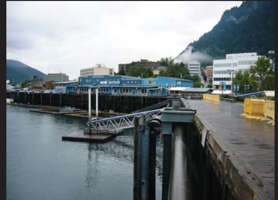
The existing dock/ seawalk currently dead ends at the lightering float, shown above. This will be removed as part of the 16B project, allowing the seawalk to continue.
