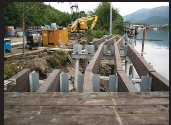
Work in progress in front of Taku Fisheries parking lot.
