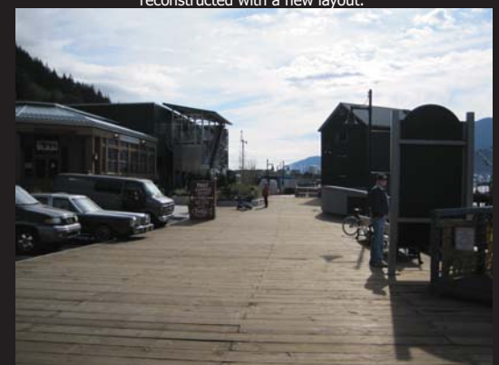
The completed seawalk approaching the Twisted Fish. Taku Fisheries new RSW fish processing system is visible in the background.
