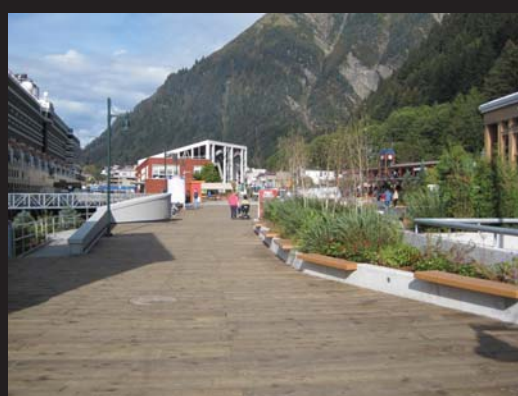
The north extent of this completed section of seawalk.
