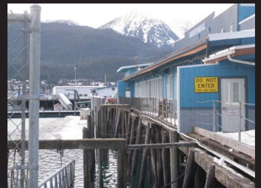
The seawalk is proposed to run along the waterside of the Merchant's Wharf building.
